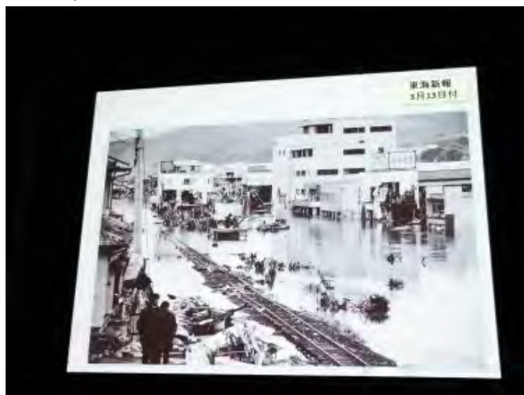
Picture showing the damage done by Earthquake & Tsunami in 2011
